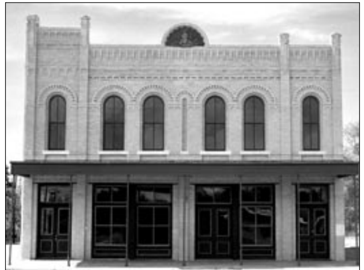
After: historically appropriate window placement
