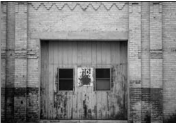
Before: note the faint outline of the original brick archway
