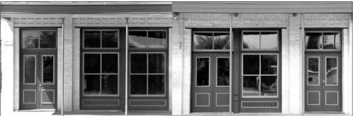
After: Removal of entrance aluminum door and restoration of doors and window in front
