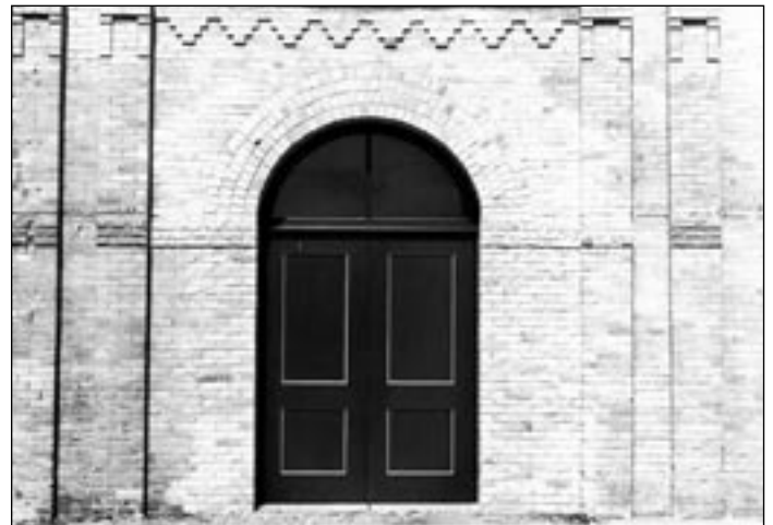
After: bricks replaced and repointed, cleared of old paint
