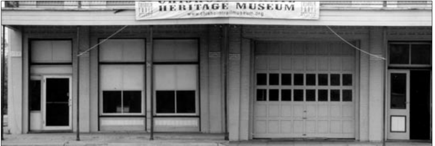
Before: Overhead garage door before restoration.
